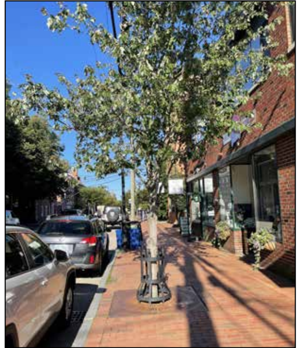
Twelve-year-old stormwater tree filter Portsmouth, NH
